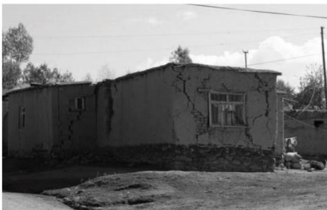
Figure 1. Earthquake damages on rural structures
