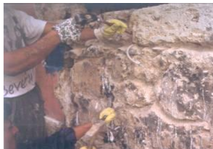
Figure 3. Re-pointing strengthening method
