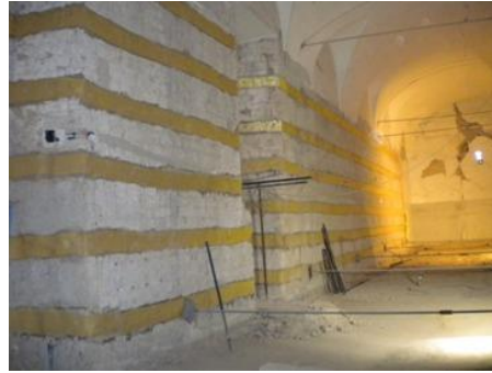
Figure 1. FRP retrofitting method
