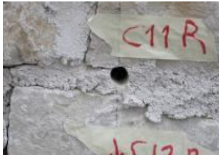
Figure 2. Grouting injections
